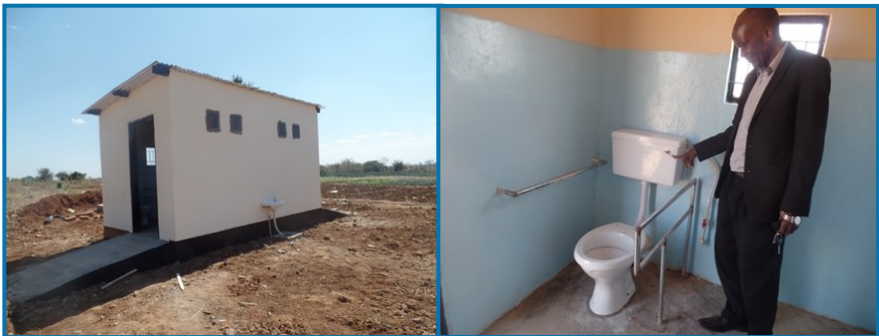
The new toilet block
