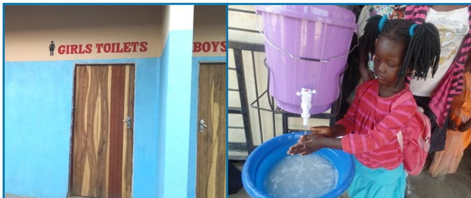
The new sanitary block
