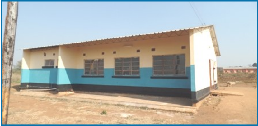
The spruced-up dormitory
